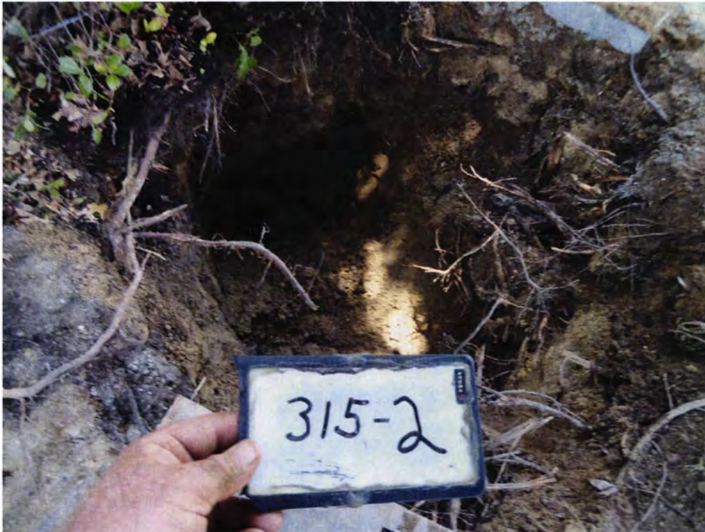
Picture 3: UST 315Ash-2 excavation.
