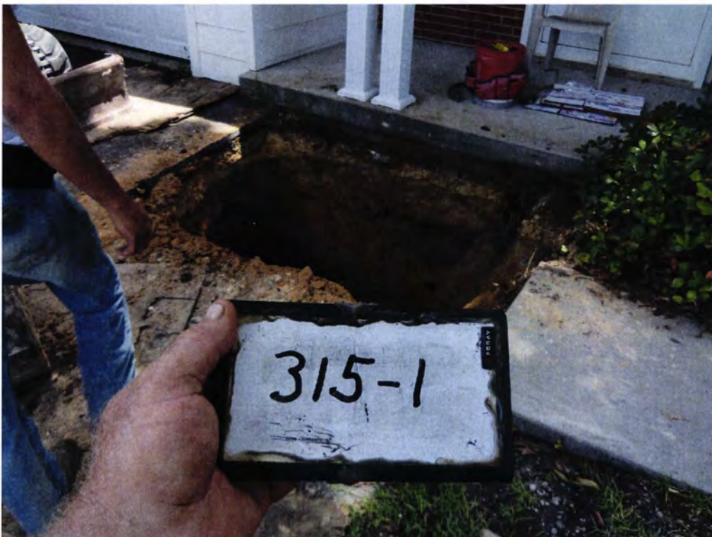
Picture 2: UST 315Ash-1 excavation.
