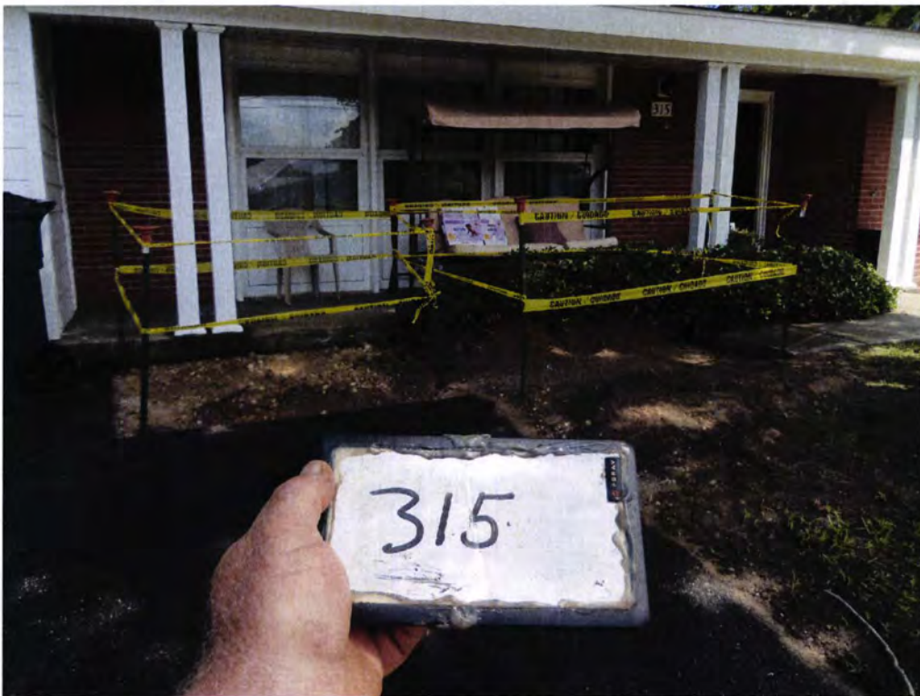
Picture 4: 315 Ash Street site near completion of work.
